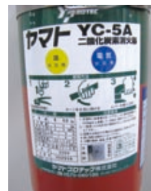
Chugai has replaced its halon fire extinguishers with CO 2 extinguishers.
