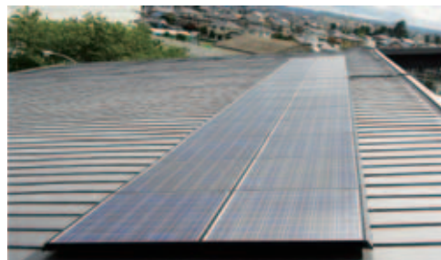
Photovoltaic panels installed on the new administrative office building of the Fujieda Plant
