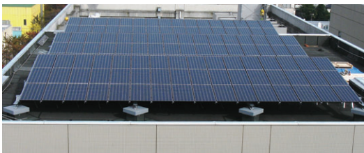
Photovoltaic power generation equipment installed on the roof of the investigational biopharmaceutical drugs wing at the Ukima Site
