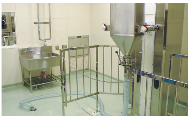
Drainage line and part of the Formulation & Packaging Pilot Plant 2
