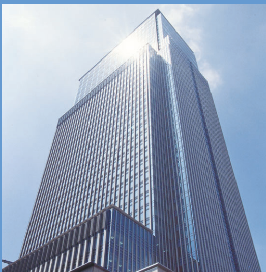
Nihonbashi Mitsui Tower (Head Office 15-20F)
